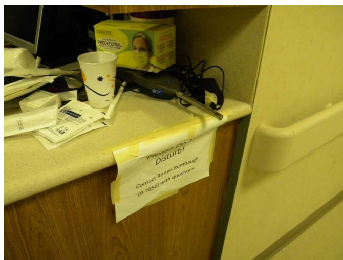
Figure 4.3: Views of the after renovation material finishes and sound level meter set-up in University Tower 6 West. (a) the nurses' station, (b) the patient room, and (c) the hallway.
